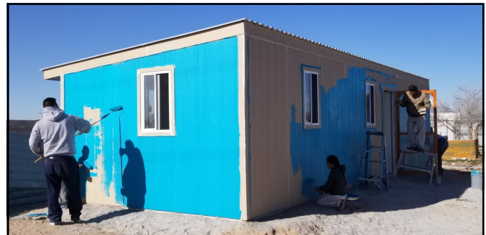
A typical team-built home, almost finished.
