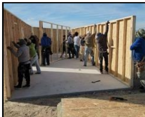
Holding up the walls
